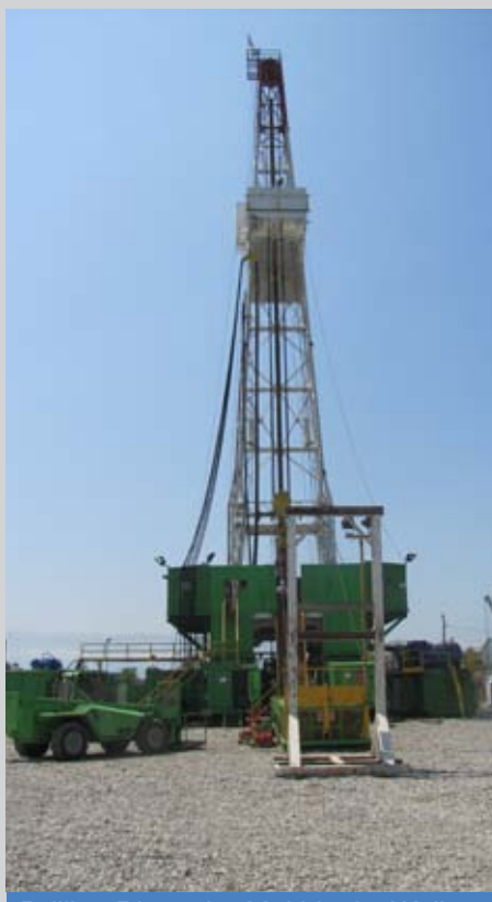
Drilling Rig at the Mukhiani 1 Well
