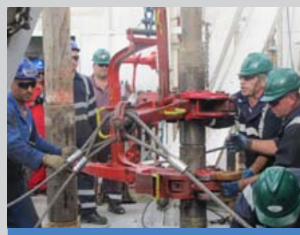
Drilling Operations in Progress
